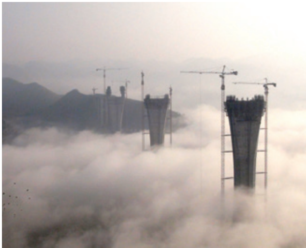
Potain tower cranes help build Chishi Grand Bridge in Hunan, China.
