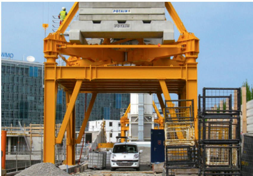
Potain cranes operate on bases that guarantee a compact footprint at the job site.
